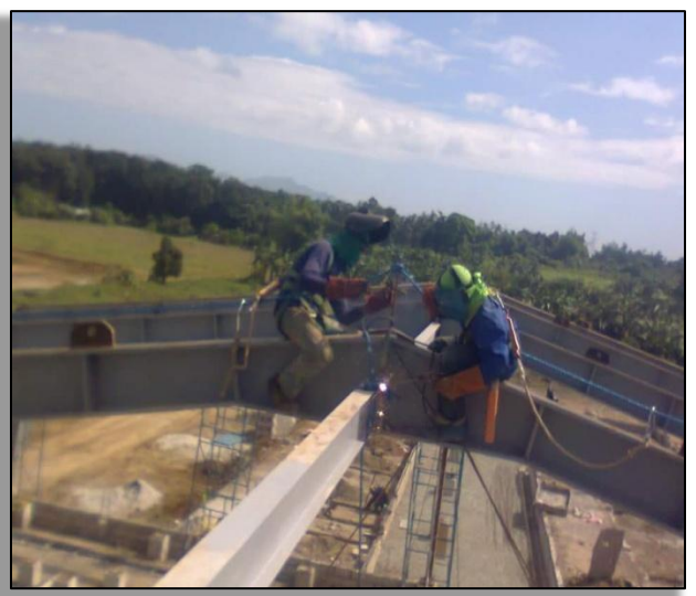
Warehouse Construction, Batangas City
