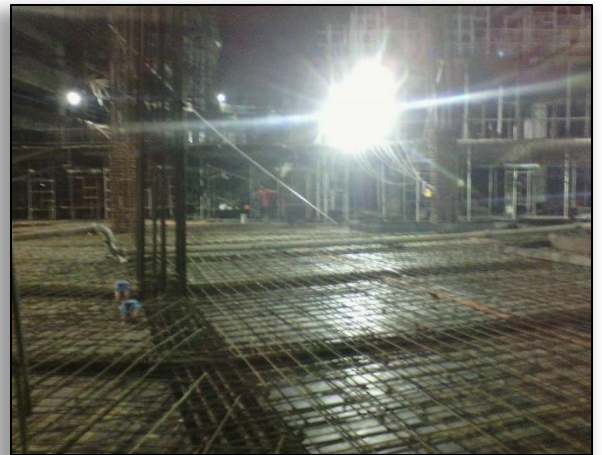
Rebar Installation, Uptown Mall, BGC
