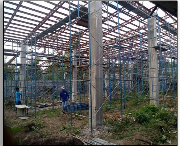
Scaffolding Installation, Kimja Warehouse, Binangonan
