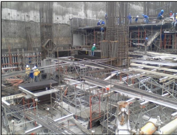
Formworks Installation, Uptown Mall, BGC
