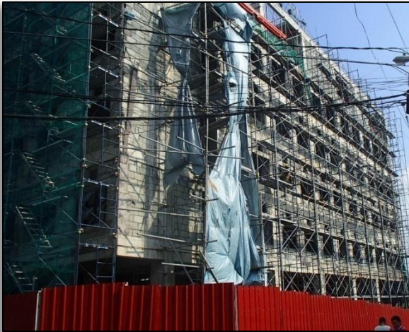
Scaffolding Installation, Newtown, Makati
