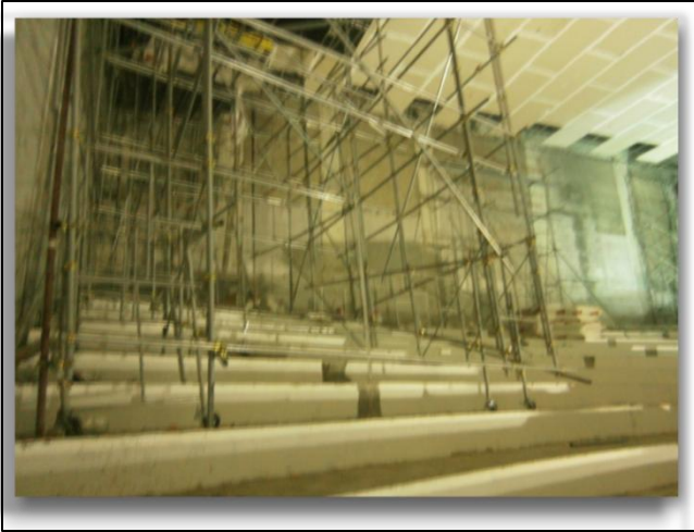
Ceiling Works, SM Cabanatuan, Nueva Ecija
