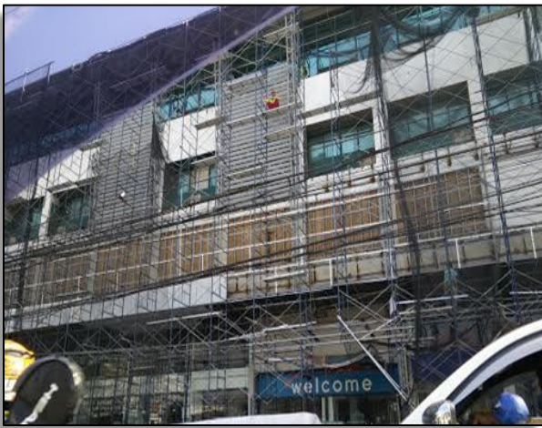
Scaffolding Installation, Mandaue Foam Facade
