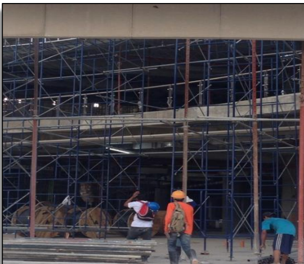
Scaffolding Installation, Robinsons Bulacan
