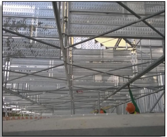
Scaffolding Installation Mama Sita's, Pasig City
