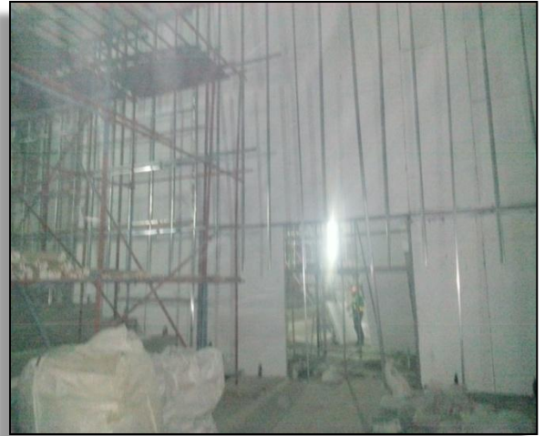
Dry Wall Installation, SM Cabanatuan, Nueva Ecija
