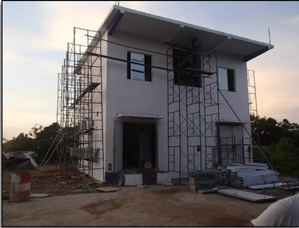
Gozar Radar Station Philippine Air Force, Lubang Island , Mindoro
