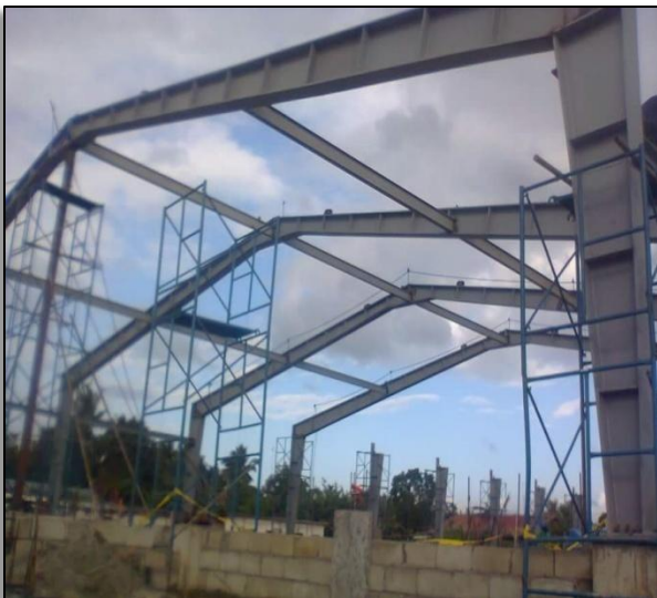
Warehouse Construction, Batangas City
